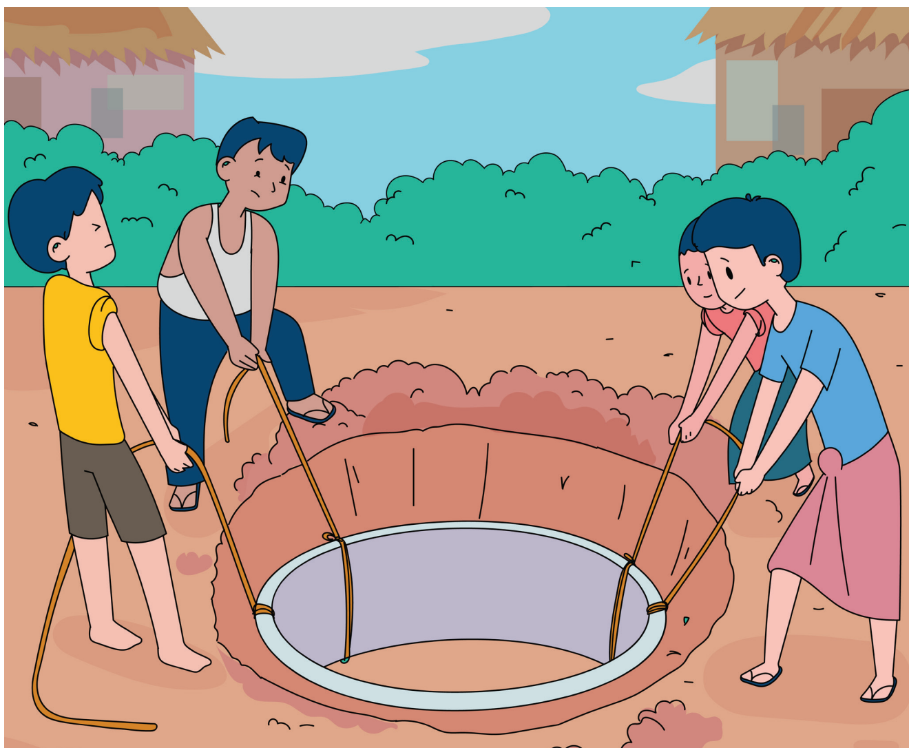
Upgrading a Dug Water Well with Concrete Rings
