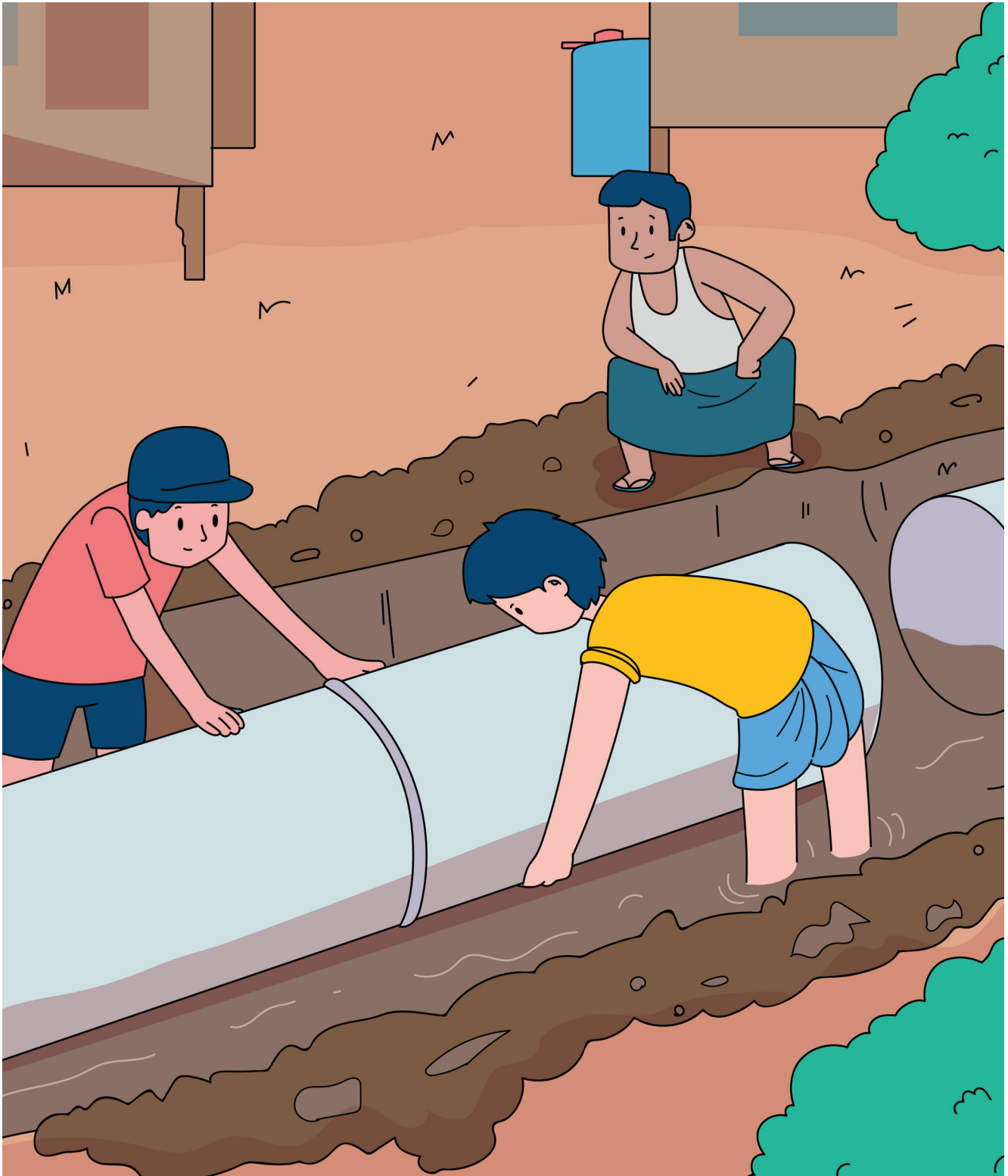
Drainage Pipe Replacement
