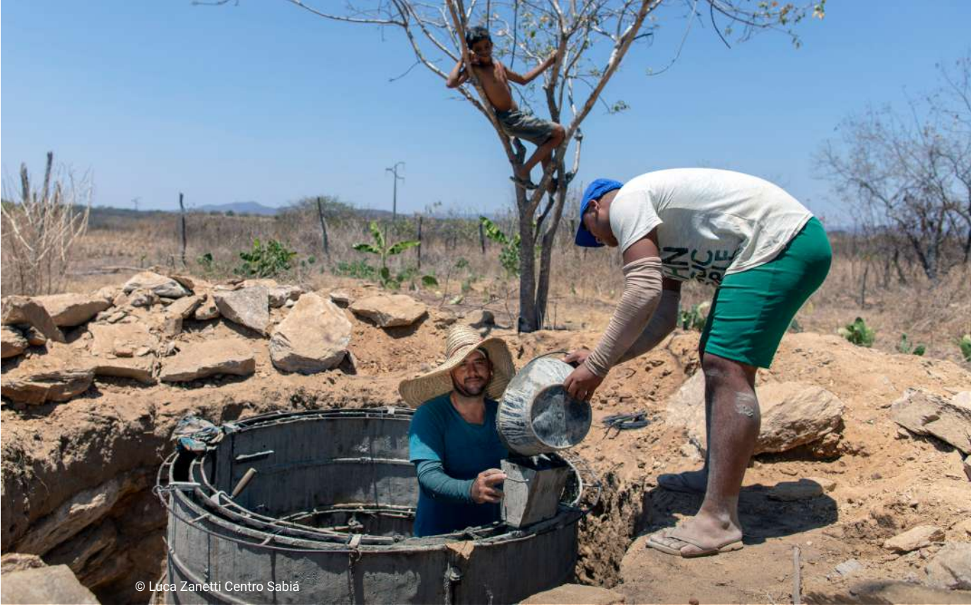
Two men installing a RAC-SAF water recycling system to sustain crops during dry seasons.
